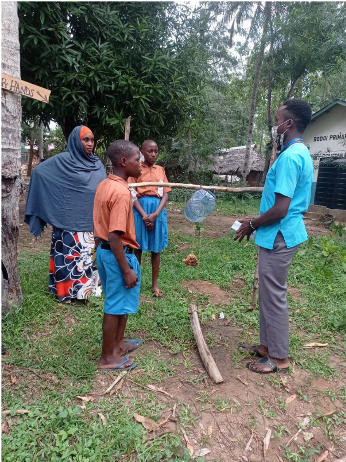
Student helps pupils to build a tippy tap installation for hand washing at the primary school in Bodoi. Photo: © Rebekah Makau
